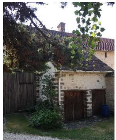
Figure 37 Exemple de descente de cave, 2018, © EG
